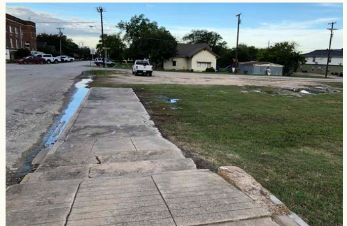
Sidewalk and drainage improvements are underway and scheduled for Downtown
