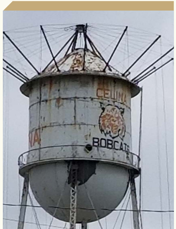
Historic water tower prior to renovation
