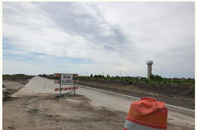
Dallas North Tollway under construction.
